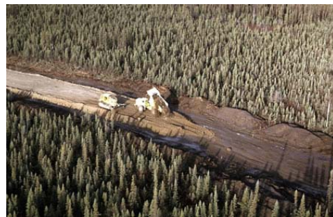
FIGURE 4.1-7 Trench Backfilling Operations (Source: TAPS 2007)
