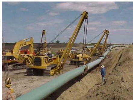
FIGURE 4.1-6 Crew Lowering a Pipeline into a Trench (Source: Photo courtesy of U.S. Pipeline, Inc. Reproduced with permission.)
