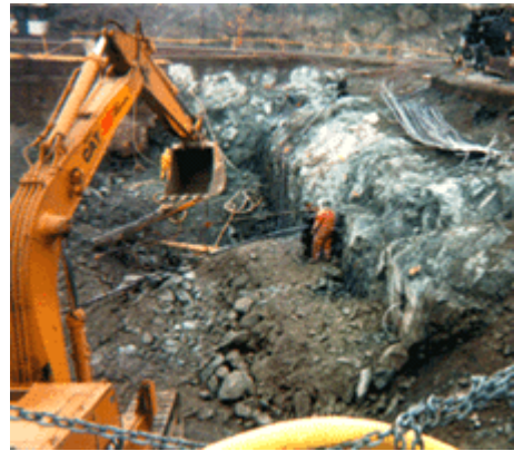
FIGURE 4.1-14 Backhoe Operations after Blasting (Source: Photo courtesy of Gulf Operators Ltd. Reproduced with permission.)
