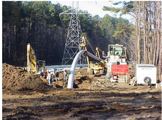
FIGURE 4.1-10 Horizontal Directional Drilling (HDD) Operation (Source: Photo courtesy of U.S. Pipeline, Inc. Reproduced with permission.)
