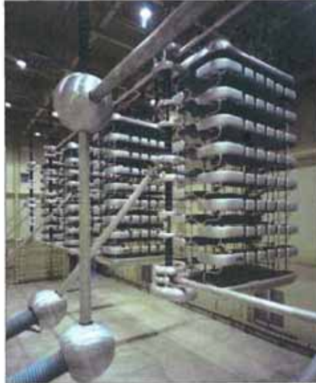
Installation of the converter stations.
