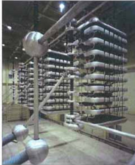
installation of the converter stations.
