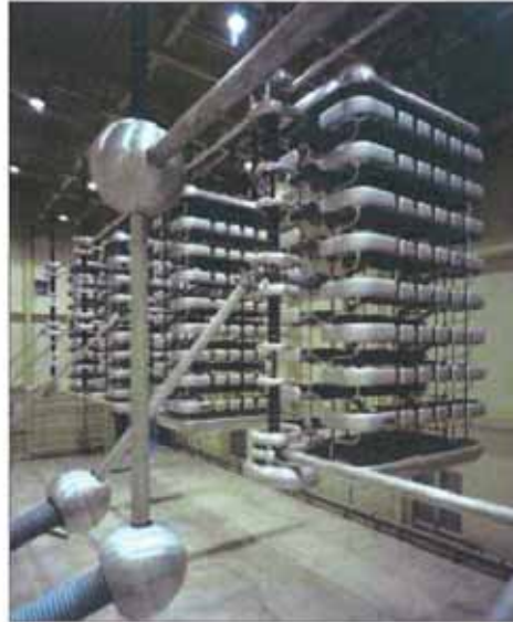
installation of the converter stations.
